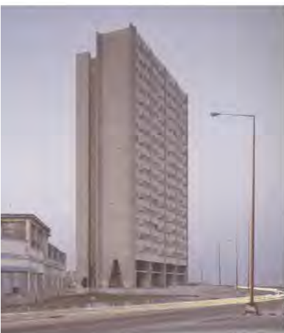
Apartment Building, A. Quintana 1967
