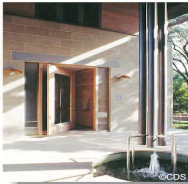
Raining Spouts + Gutters
